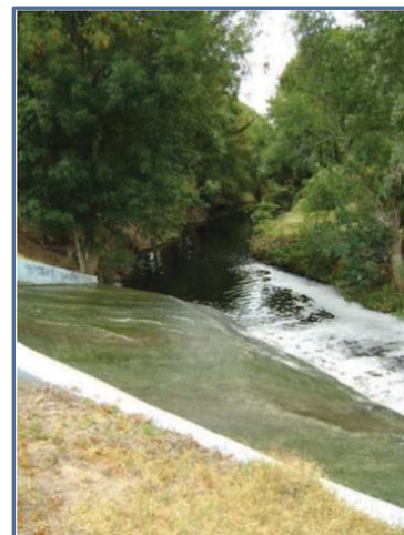
Good practice: Paving at point of discharge helps prevent stream bank
