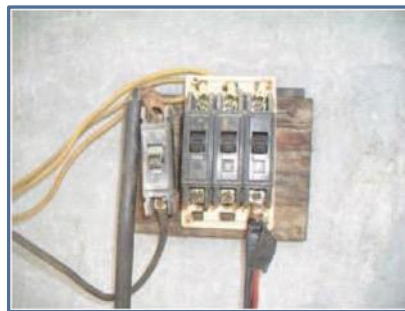
(IA) Circuit breaker with exposed and damaged wiring! Circuit breakers must be labeled and enclosed.
