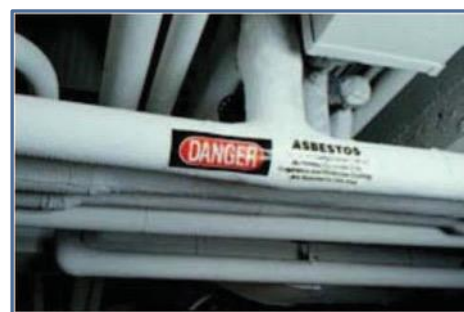
Good Practice: Asbestos-coated pipes are properly marked.
