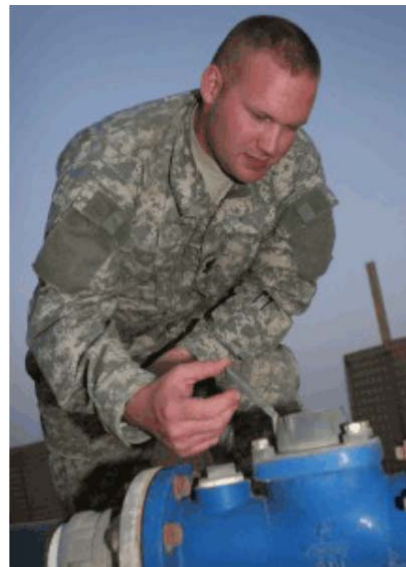
Good practice: Measure influent and effluent with flowmeters attached to incoming water and outgoing wastewater pipes.
