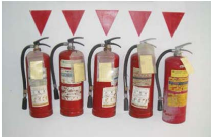
Good practice : Fire extinguisher types for potential hazards are provided and tagged
