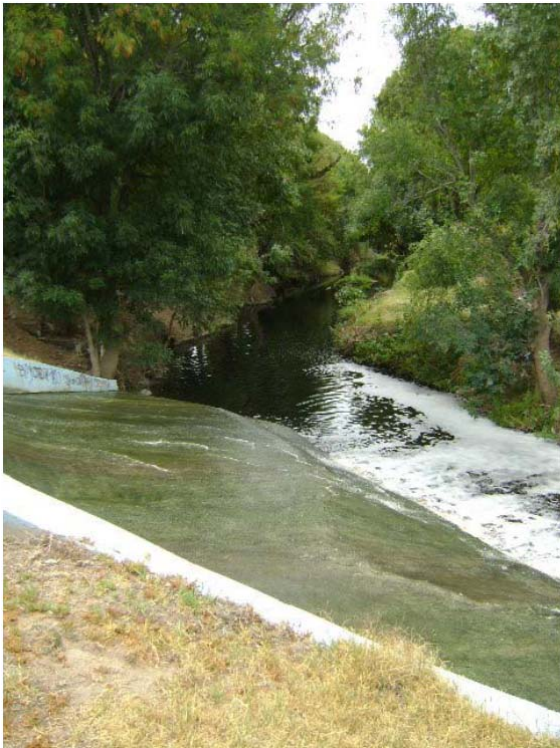
Good practice: Paving at point of discharge helps prevent stream bank erosion.
