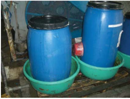
IA Bad Practice: Secondary containment is too small for these chemical drums
