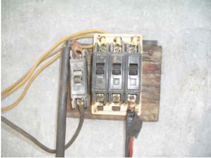
IA Circuit breaker with exposed and damaged wiring! Circuit breakers must be labeled and enclosed.
