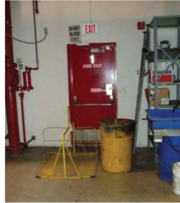
IA Bad Practice : Fire exit is blocked by trash container and equipment
