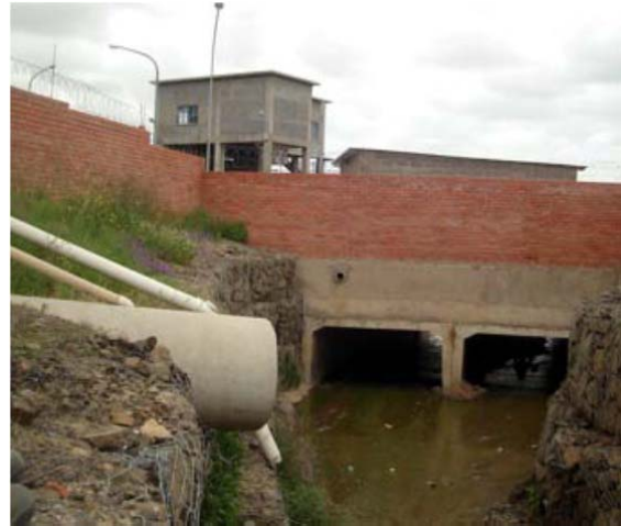
ZTV Bad Practice: Factory wastewater must not bypass wastewater treatment.
