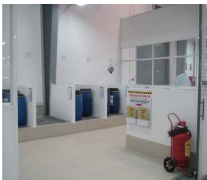
Good Practice: Chemicals stored in designated area. Area is clean and housekeeping is good.
