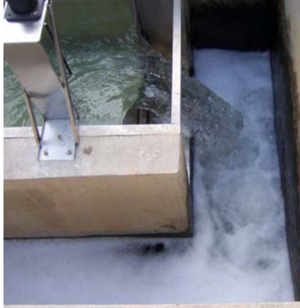
At effluent discharge points, foam should dissipate quickly. It must not persist and there should be no floating solids.
