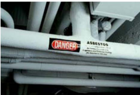
Good Practice: Asbestos-coated pipes are properly marked.
