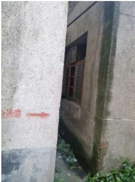
Picture 30: In Zhiqiang, the fire exit is so narrow that only one person could pass by.
