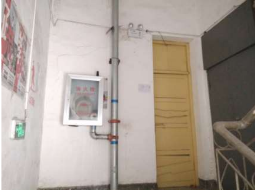
Picture 29: In Zhiqiang, the door supposed to be fire exit was locked and couldn't be open.
