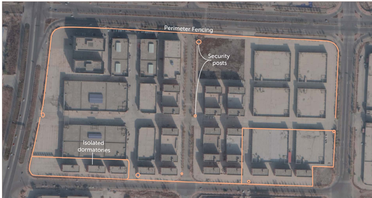
Figure 11: Satellite image of HYP’s factory in Shule (Yengixahar) county, Xinjiang
