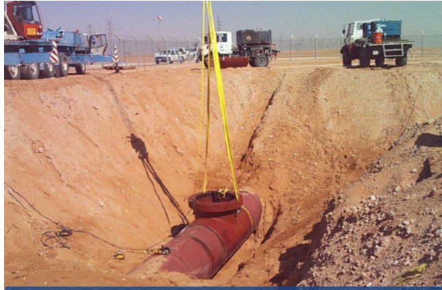
A Saudi Aramco oil pipeline upgrade in Saudi Arabia.
