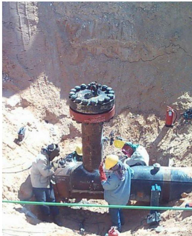
Migrant workers on a crude oil pipeline upgrade project for Saudi Aramco. They told Equidem that their employer, an Aramco sub-contractor, terminated their contracts after the COVID-19 pandemic started. The men say they are owed wages and their end of service benefit payments. © Equidem 2020.
